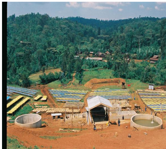
Fig-7 Large scale wet coffee berry processing plant.
