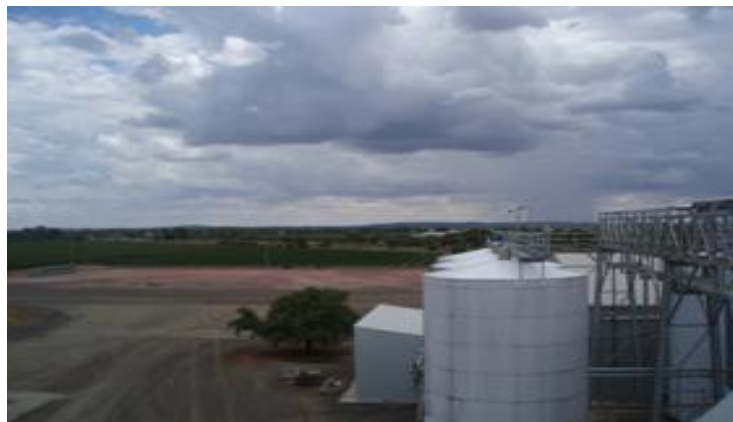
Fermentation Wine Tanks near Yenda NSW – Photo by Grant Pettrie
