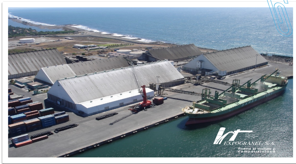
Figure 3 EXPOGRANEL Facilities at Port Quetzal
