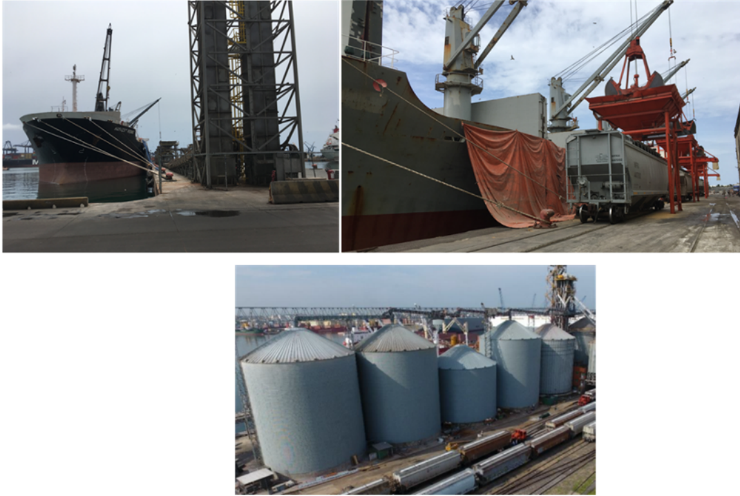
Fig. 18 Grain terminal and internodal rail yard inside the Port of Veracruz.
