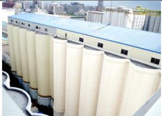
The biggest silo facility in the Chiba port consists of a total of 253 bins divided by 4 control towers. Chiba Kyodo Silo Co., Ltd.
