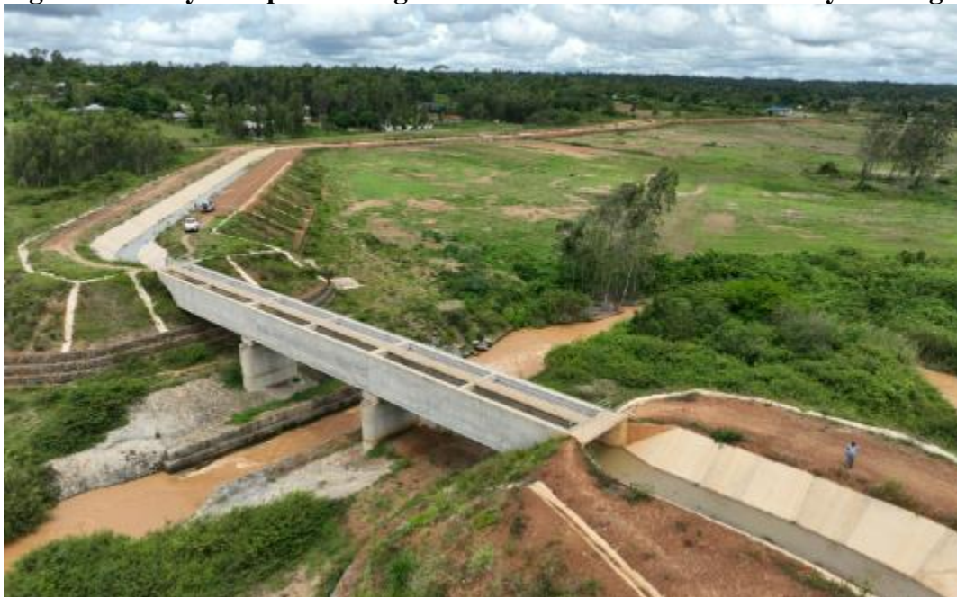
Figure 8: Newly Completed Irrigation Canal Infrastructure in Bunyala Irrigation Scheme
