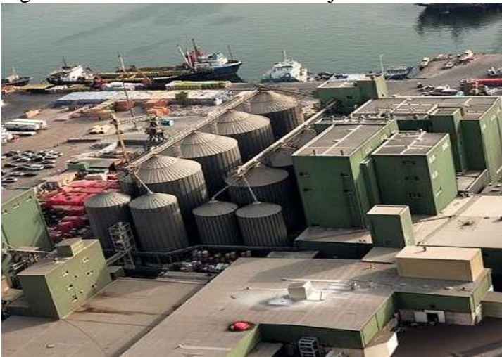
Figure 6: IFFCO Grain Silos at Sharjah Port
