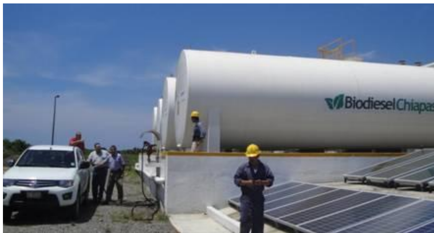
Ag Minister Counselor Dan Berman operates the pump at the biodiesel plant in Puerto Chiapas.
