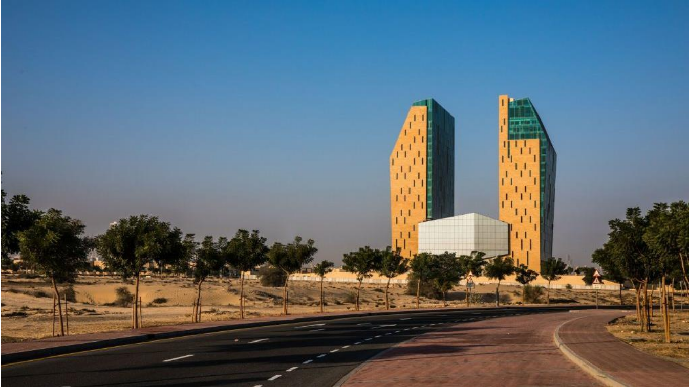
The Recently Completed Dubai Science Park Towers
